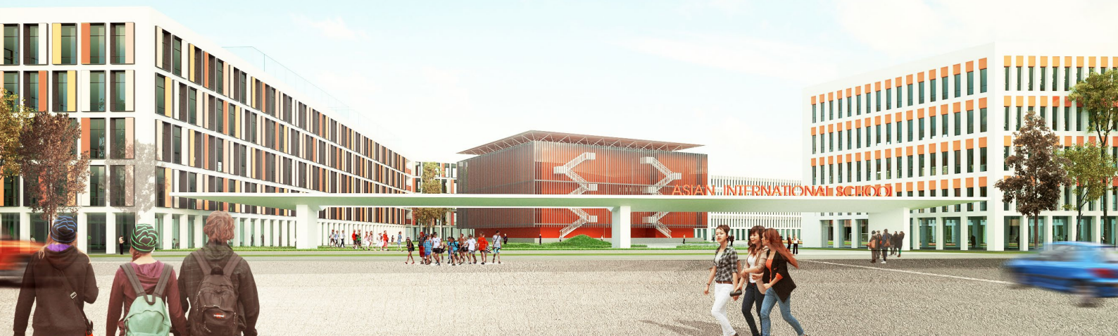
ASIAN SCHOOL PROJECT in Sonky Ward, Tanphu District, HCMC
