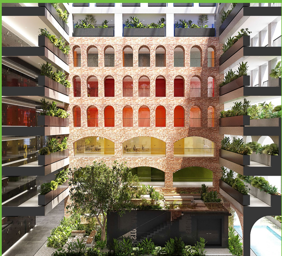
ASIAN SCHOOL PROJECT in Tangnhonphu Ward, Thuduc City, HCMC
