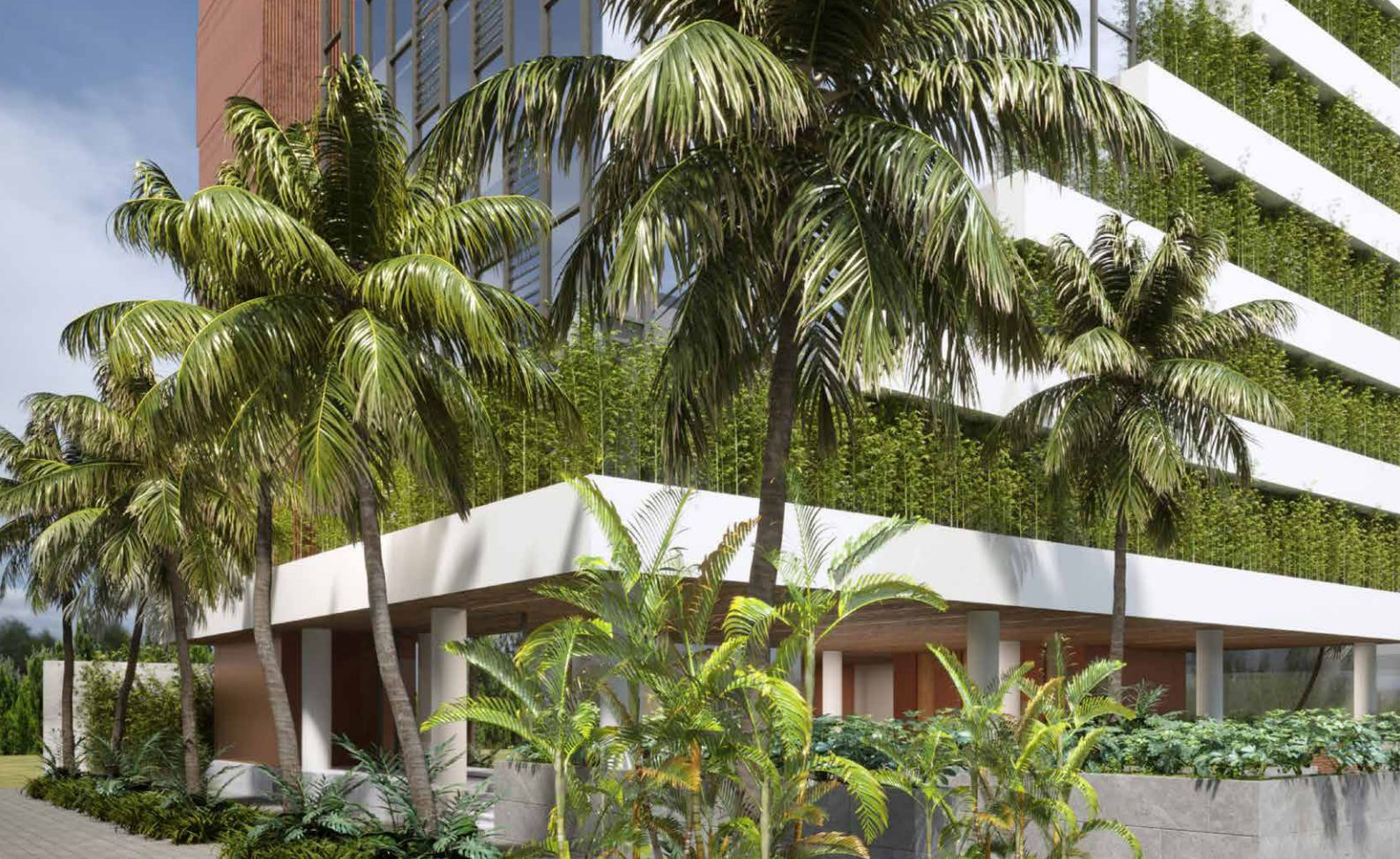
SIU PROJECT (under construction) in Thaodien Ward, Thuduc City, HCMC
